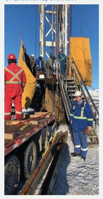
RMSPumptools was selected to provide 'packer penetrator systems' at the Clive Field in Alberta, to protect the oil well casing from the potentially damaging effect of the captured CO<sub>2</sub>.
